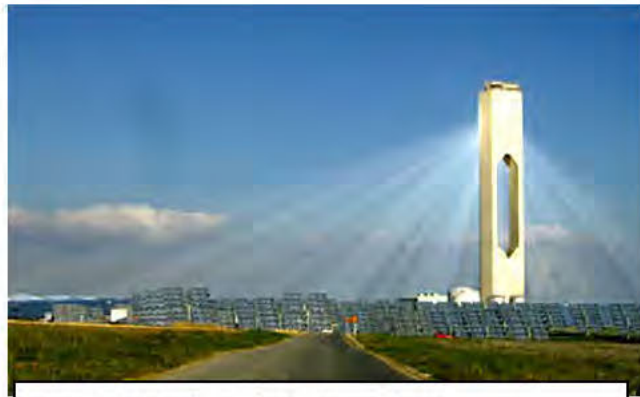
Figure 8: Seville solar power facility ( http://inhabitat.com/sevilles-solar-power-tower )
